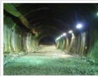
Waterway tunnel construction
