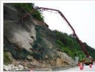
Excavated slope reinforcement construction
