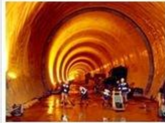
Subway tunnel construction
