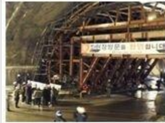
Highway tunnel construction
