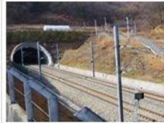
High-speed railway tunnel
